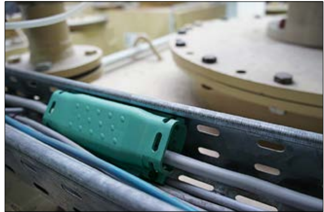
Gel cable joint Relifix V in use as a cable repair.
