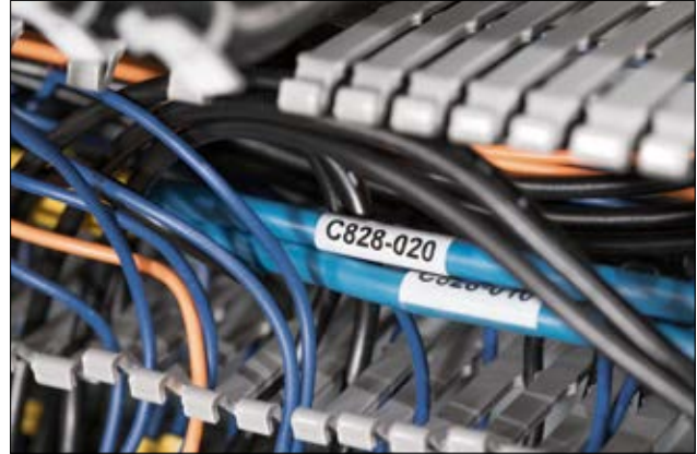
Helatag 896 offers an excellent protection against abrasion and environmental impact.
